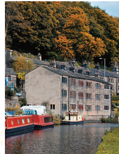
ROCHDALE CANAL – HEBDEN BRIDGE
